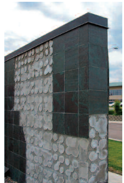
Picture 1. Adhered veneer failure. Materials used must be durable for severe weather application. The durability of an adhered veneer used in Sedona, AZ is different from that for a product used in the Midwest with wind driven rain, water penetration and freeze/thaw cycles.
