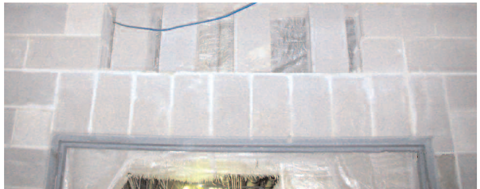
Figure A. Non-modular (2" trim) standard hollow metal frame with cut units
